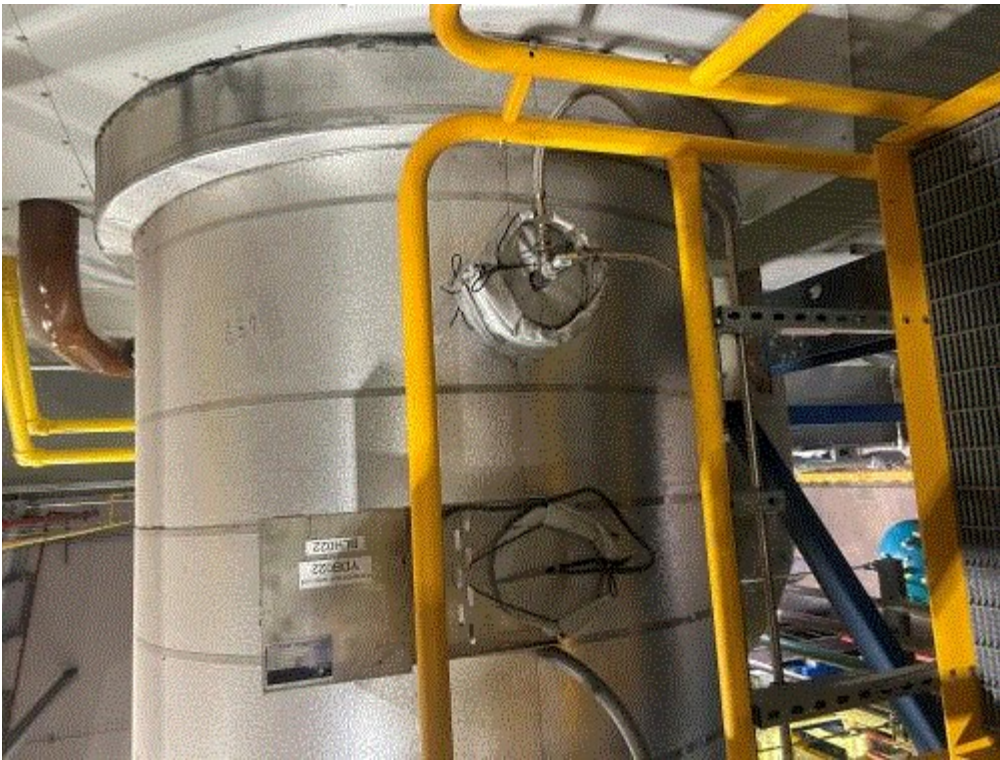
Image 2(Urea inlet) : Inlet for the urea fluid for EURICE 2
