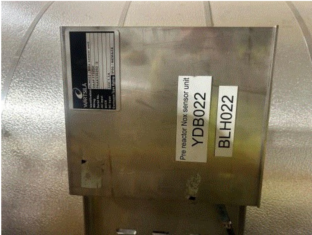
Image 4(NOx sensor unit) : Pre reactor NOx sensor unit for EURICE2
