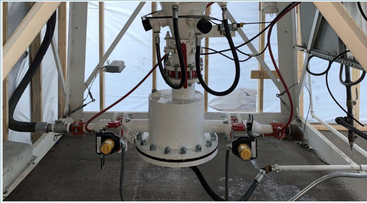
Graphic 2 – DSI Reagent Injection System Piping
