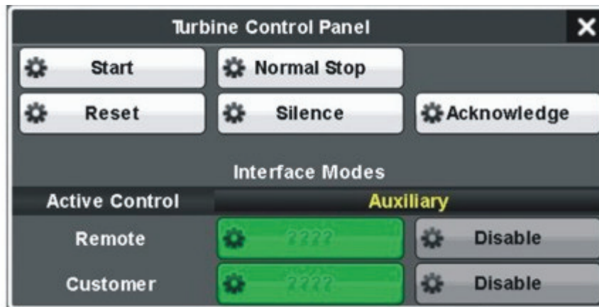
Figure 3.1.7 Onscreen Turbine Control Panel
