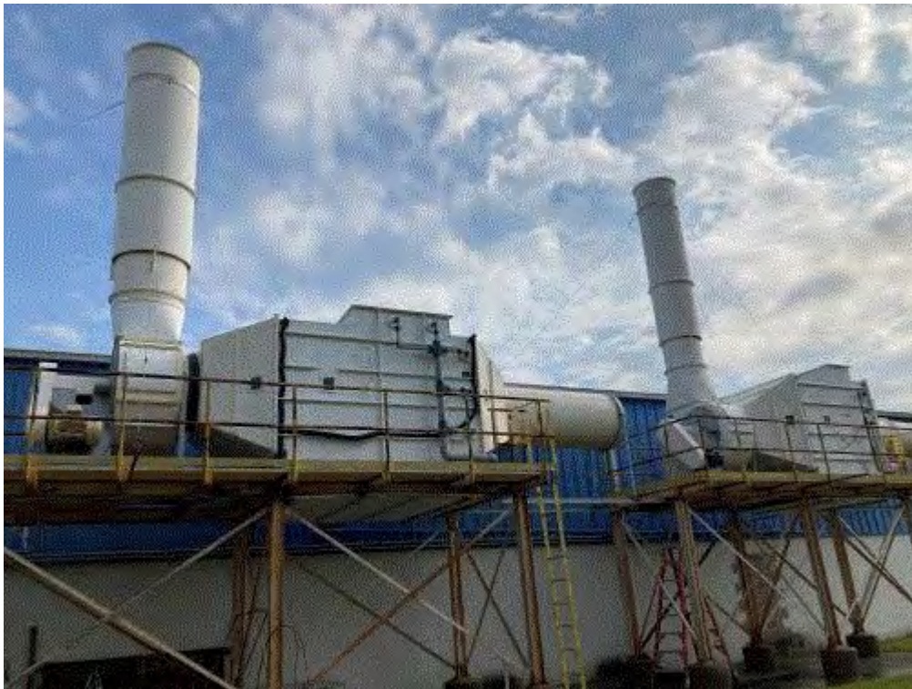
Image 2(Stacks) : Alkaline and acid scrubber stacks. No opacity noted.
