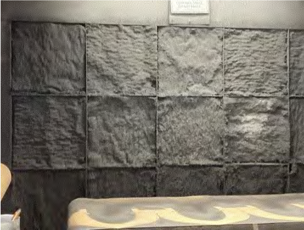
Image 3(Coating Booth) : One of 2 coating booths. Note gaps in filters along edges of each square.
