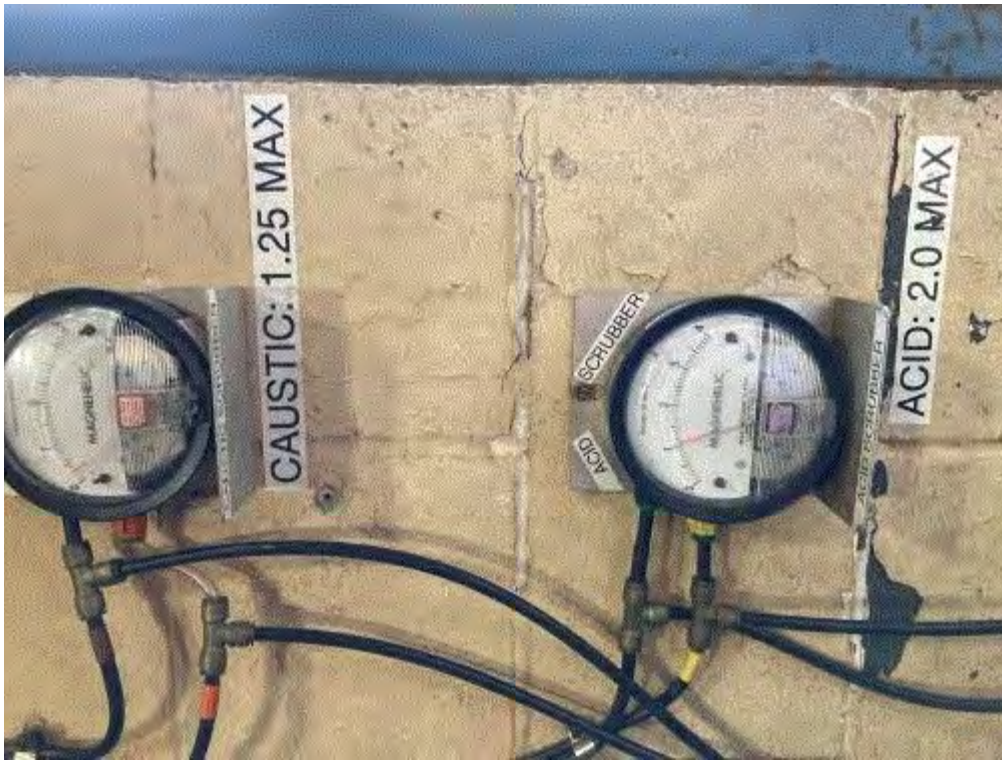
Image 1(Pressure Drop) : Monitors used for pressure drop and alkaline and acid scrubber systems.
