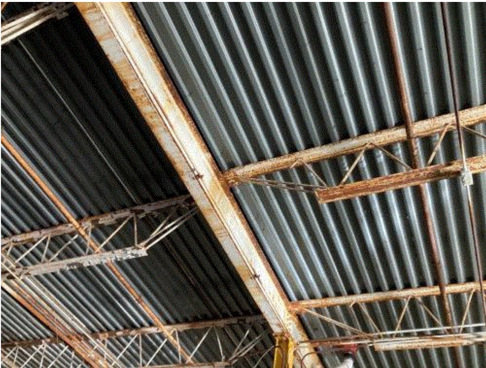
Image 2(Roof 2) : Image of the new roof in the south portion of the facility.
