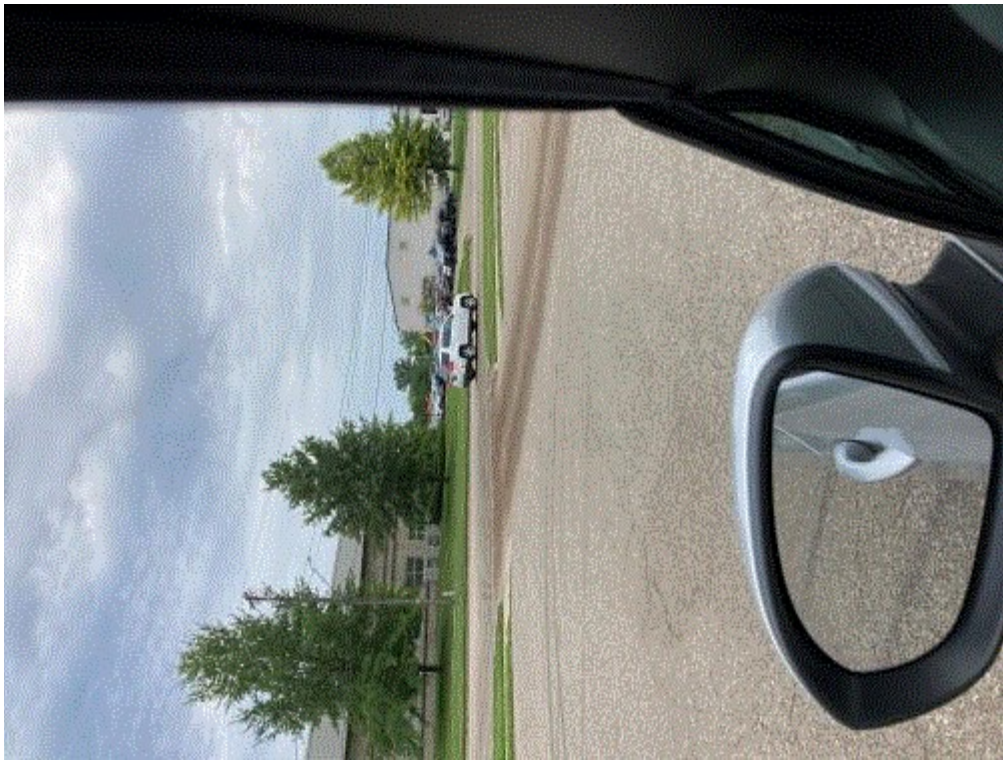
Image 9(Track out) : Track out observed from truck traffic exiting the northernmost roadway. 8/23/23
