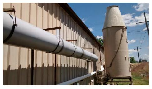
Photo 2: View of scrubber for the nickel plating process and its ductwork, and the south exterior wall (2016).
