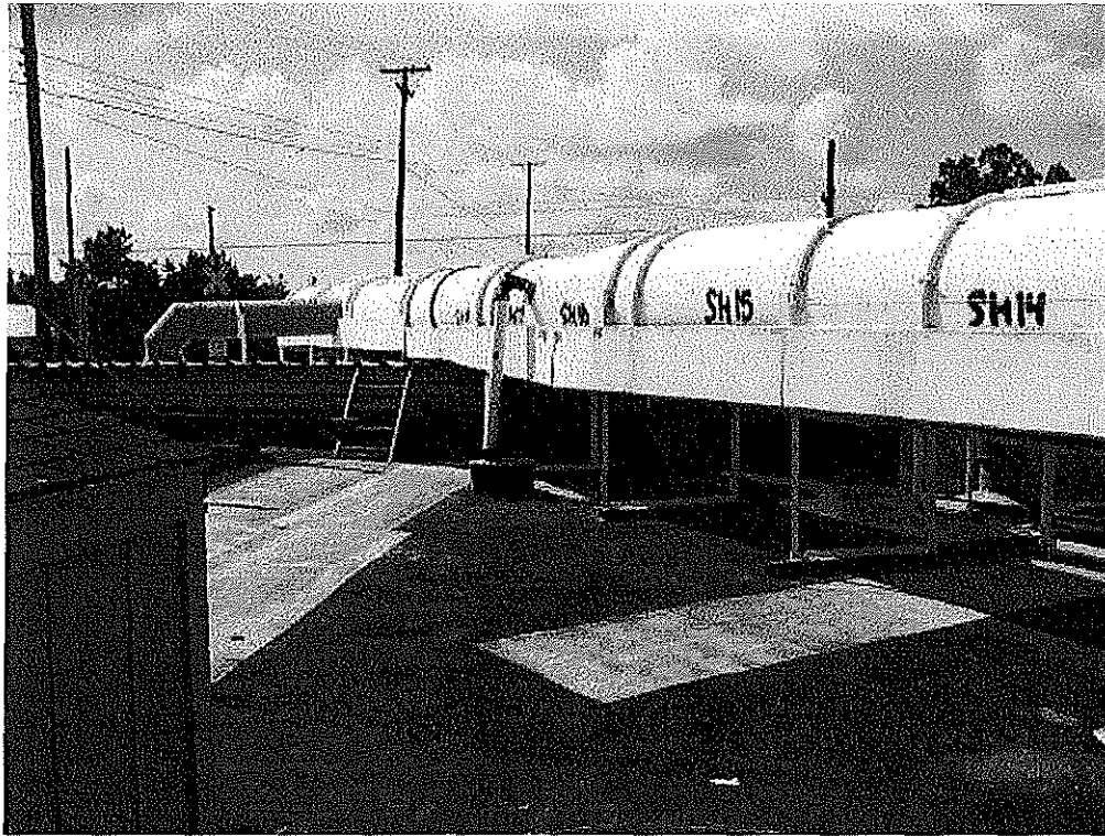
Image 4(004) : West ductwork on east roof, looking south.
