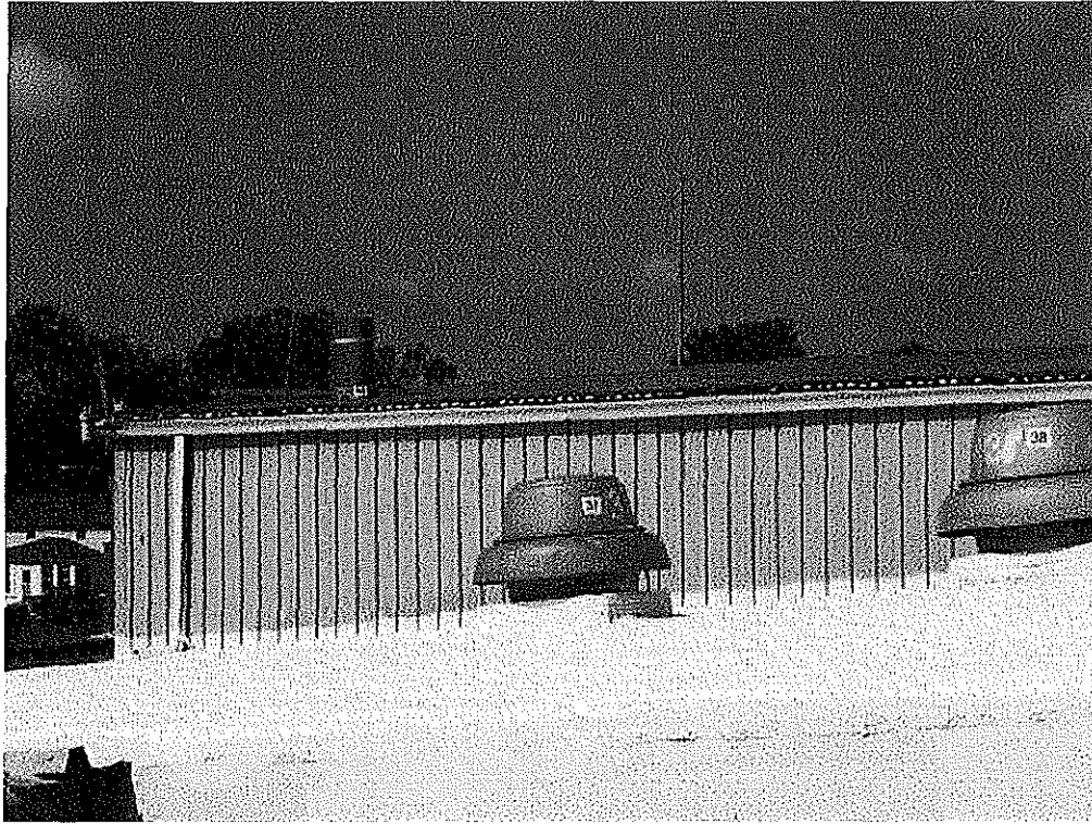
Image 8(008) : 8/30/2017 photo of taller cadmium scrubber stack, at left.
