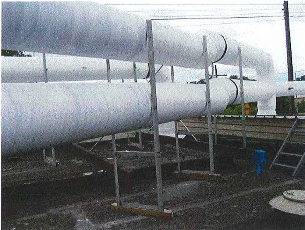
Image 3(3) : Ductwork in primer.
