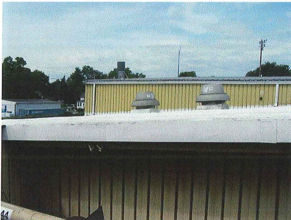
Image 10(10) : Cadmium scrubber stack (in background).
