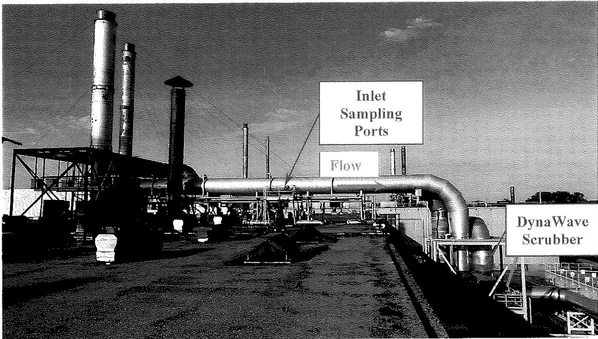
**Figure 2-1. No. 1 Biofilter Inlet Sampling Location**
