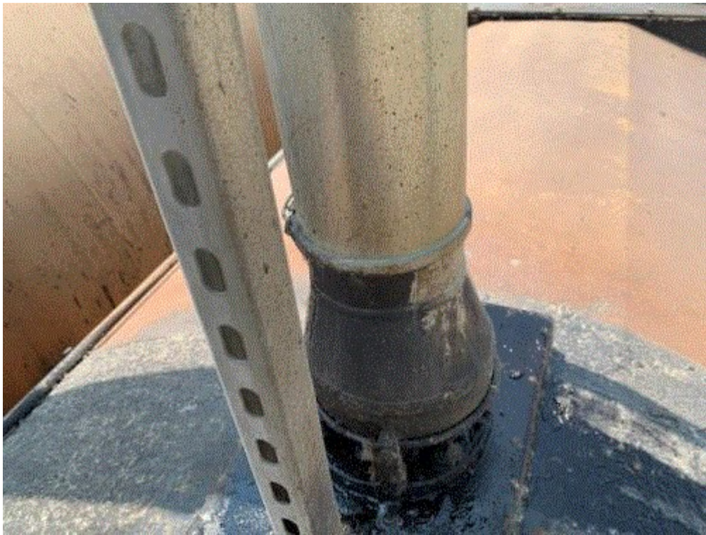
Image 1(Top of AC Tank) : Pickup point for vapors leaving AC tank to route to vapor condenser.
