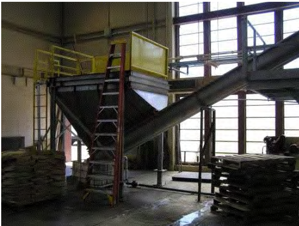
Image 5(005) : Feed hopper and auger.
