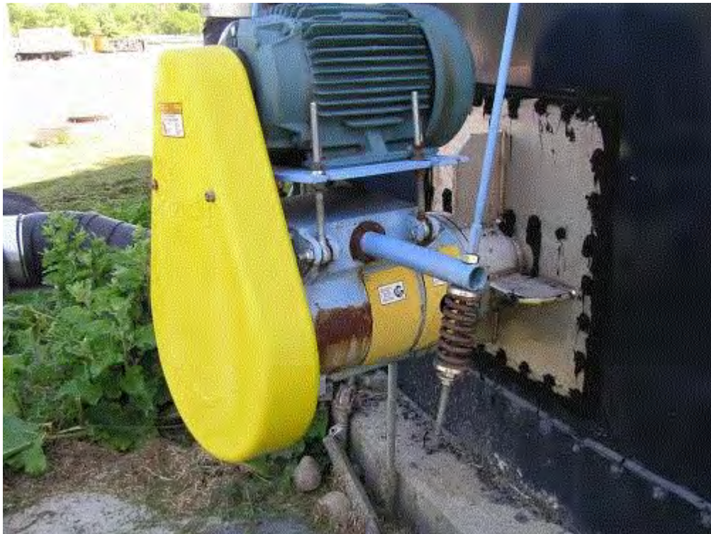
Image 3(003) : New stainless steel plate with gussets.
