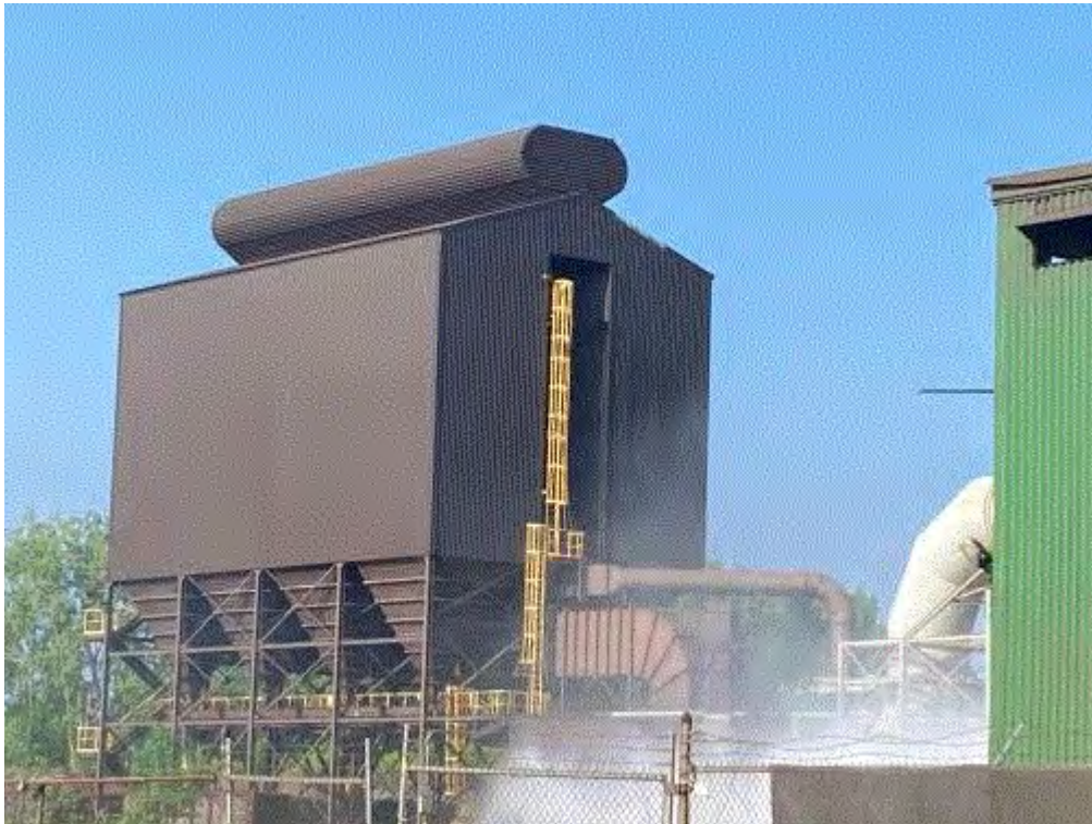
Image 1(EAF Baghouse) : EAF Baghouse
