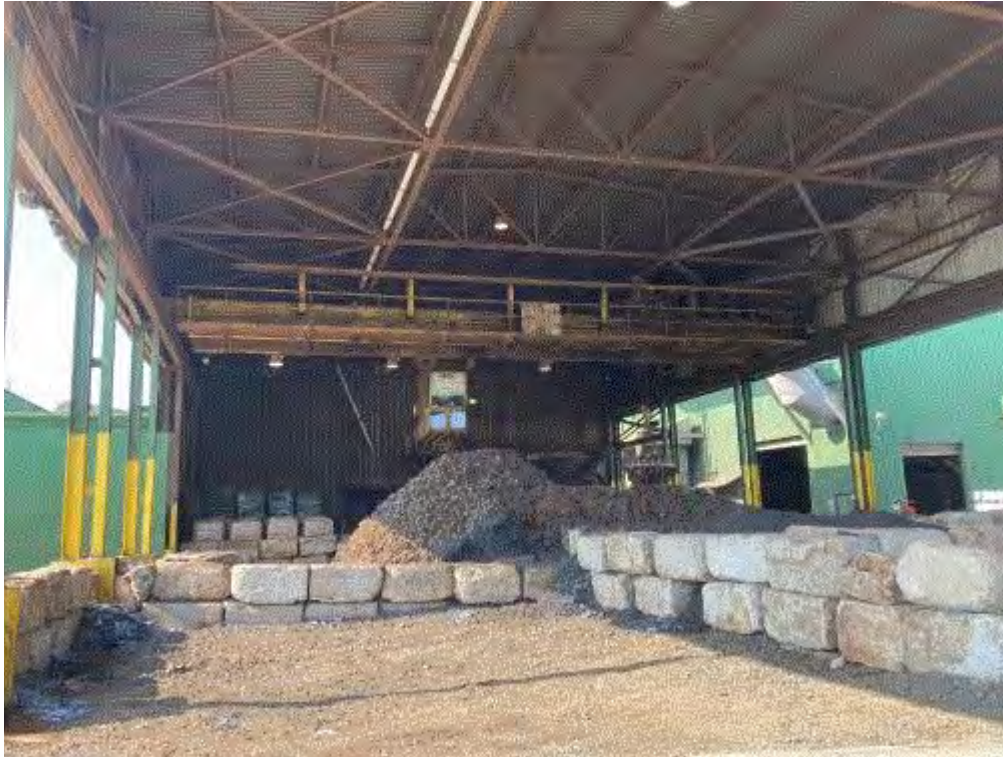
Image 8(Scrap yard building) : Scrap yard building
