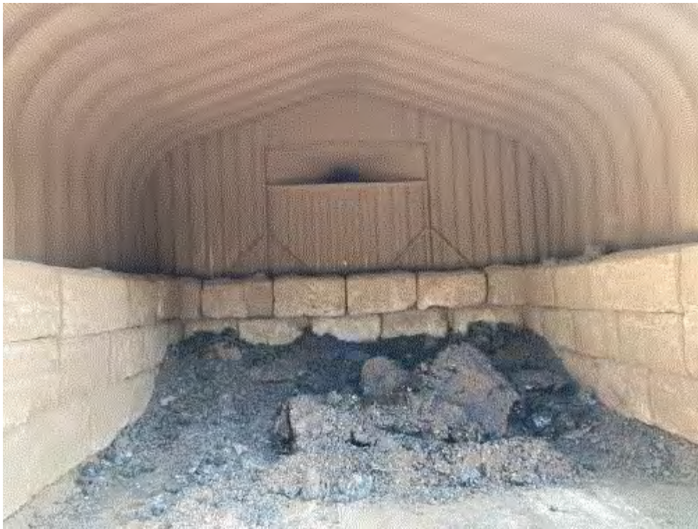
Image 9(North scrap) : North scrap pile building with vent in back
