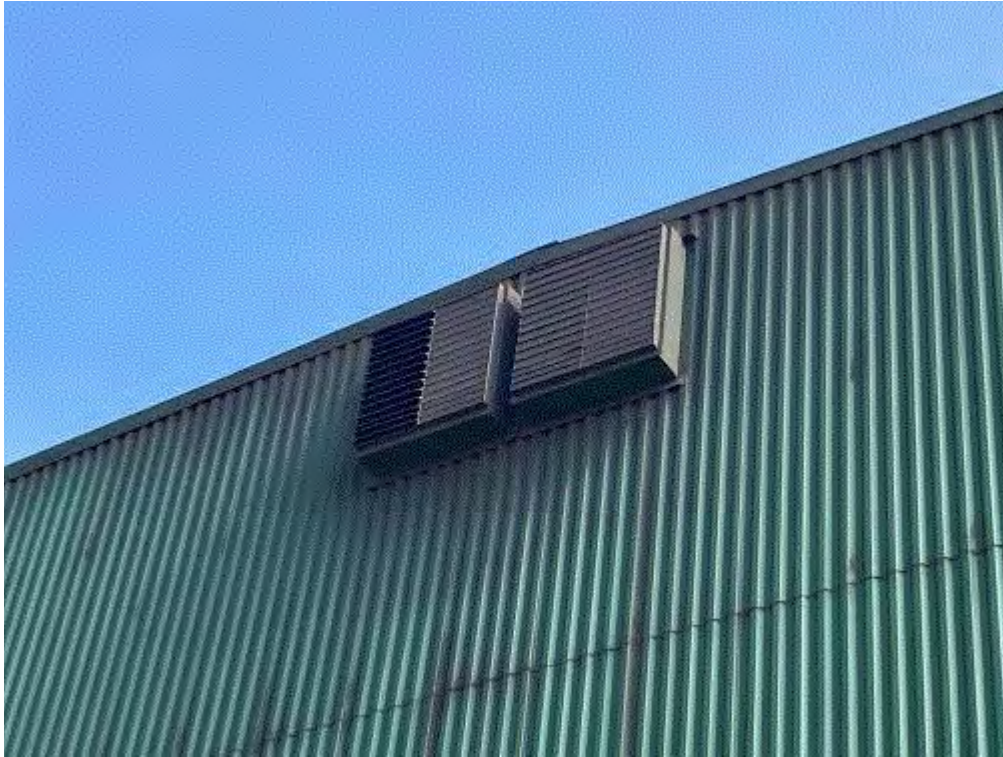
Image 11(South Vent) : Vent on southside of Melt Shop. Louver stuck open on the left(west) side of it.
