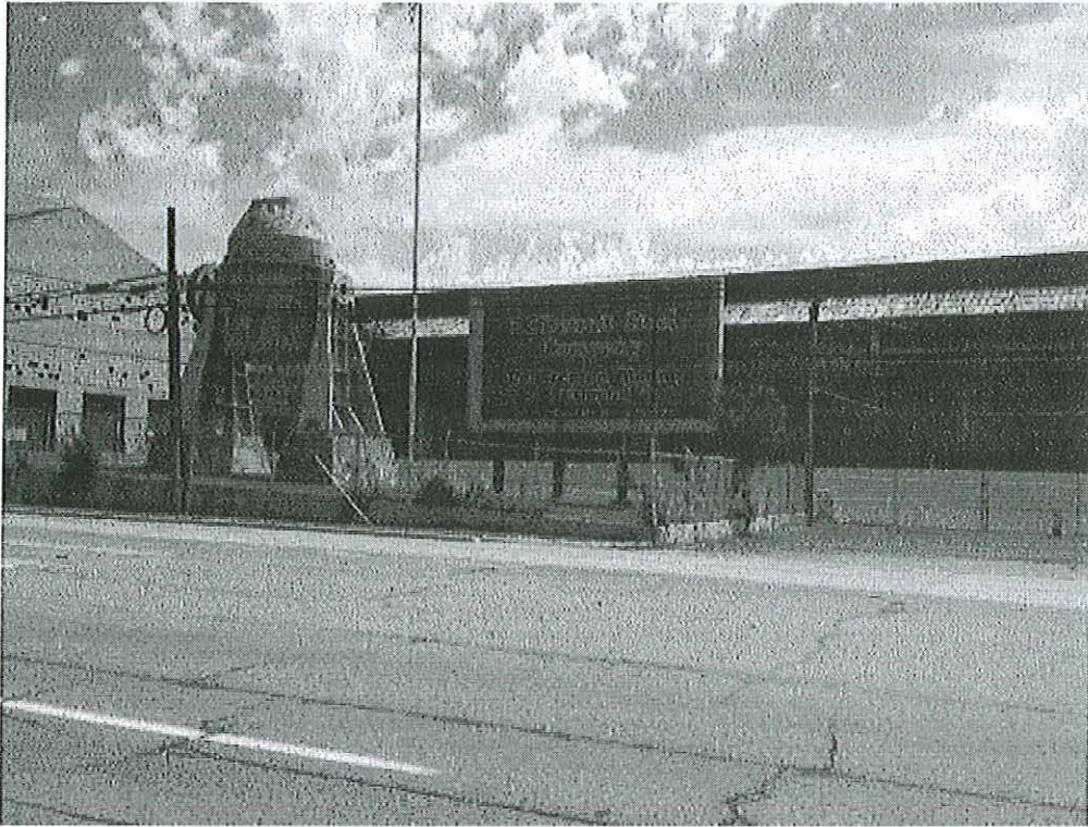
Image 1(DSC Trenton Plant) : DSC Trenton Plant/Trenton Marine Terminal front entrance.
