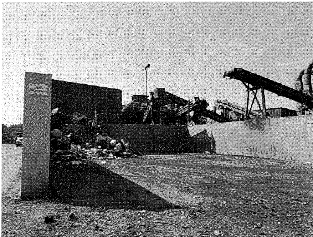
Image 14(Fluff bunker) : Fluff bunker
