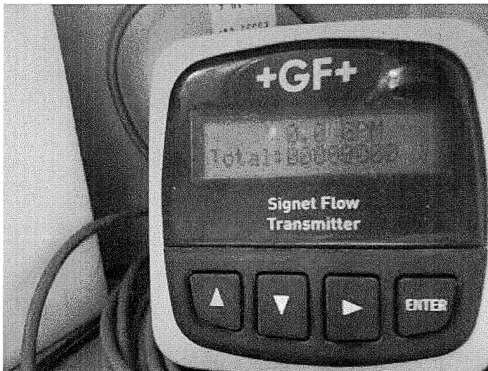
Image 16(flow rate gauge) : Venturi scrubber flow rate gauge
