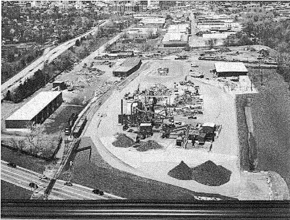
Image 1(Aerial photo) : Aerial photo
