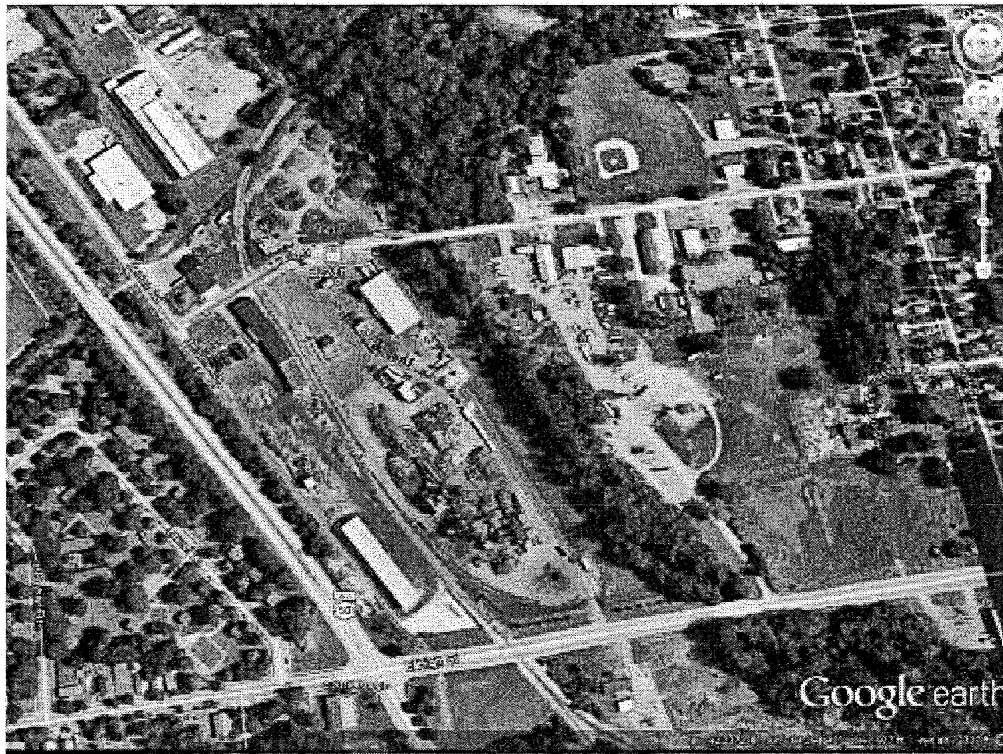
Image 1(Aerial photo) : Aerial photo of Omnisouce
