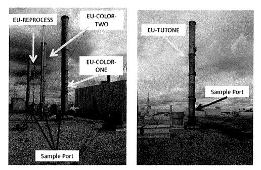
**Thermal Oxidizers (TO) Outlet Locations**
