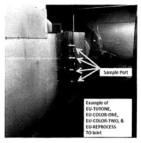
Example of Thermal Oxidizers (TO) Inlet Locations
