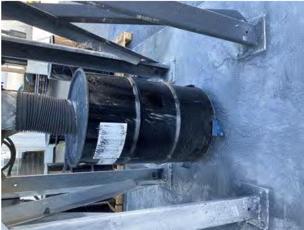
Image 8(Zinc collection) : Note particulate near base of collection drum for the zinc shot blasting baghouse.
