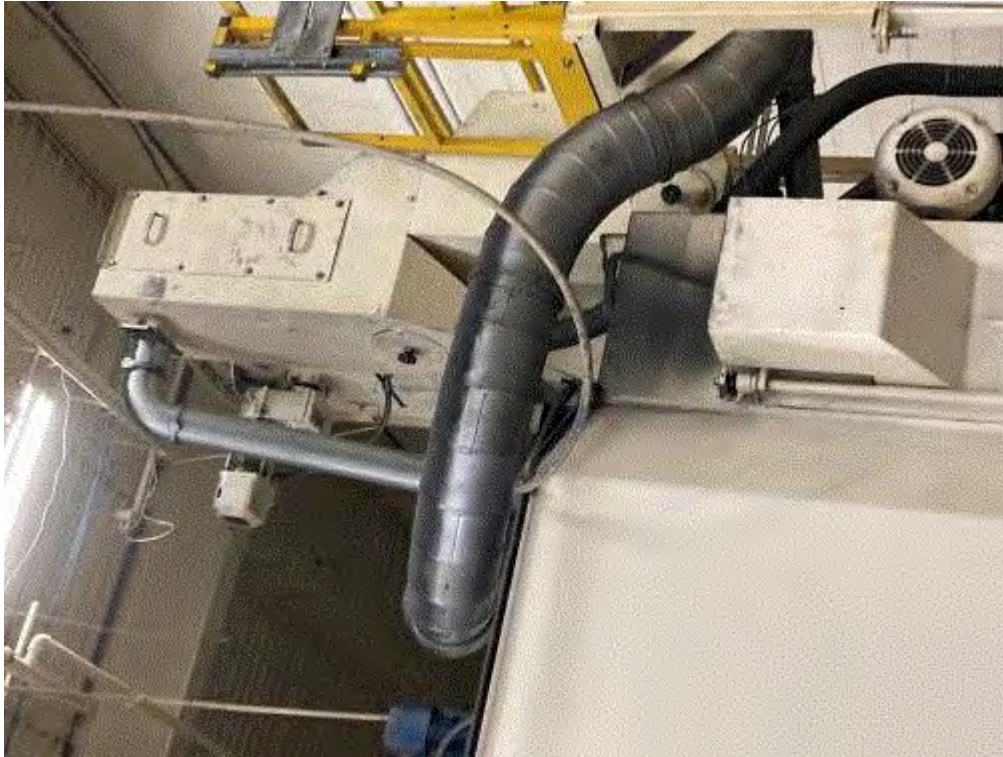
Image 6(Zinc Shot Blast) : Indoor view of ductwork leading outside to baghouse. Note the black particulate underneath the ductwork.
