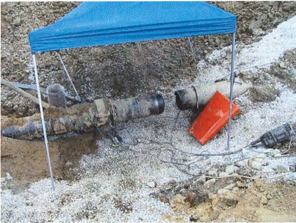
Image 2(004) : Air-gapped line, and trench.
