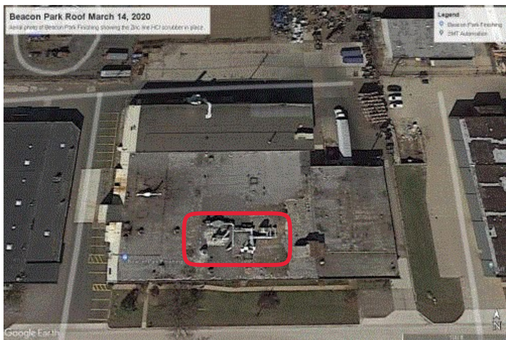
Image 1(March 14, 2020) : Shows Control B installed on March 14, 2020
