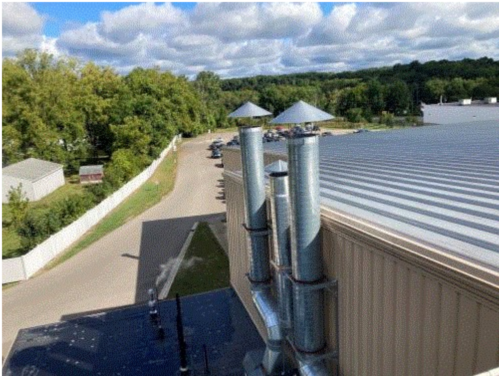
Image 2(Autoclave Oven) : 2 larger stacks from steam autoclaves. Smaller stack from hood above oven. Rain caps on all.
