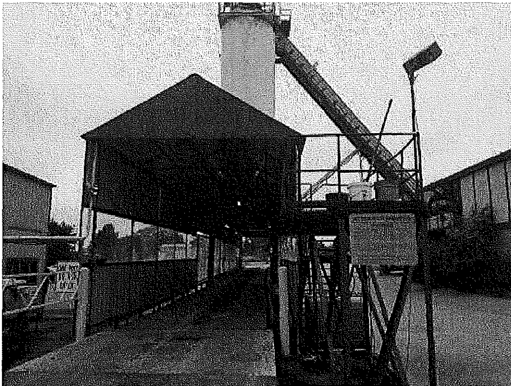
Image 2(Asphalt Loading) : Asphalt loading.
