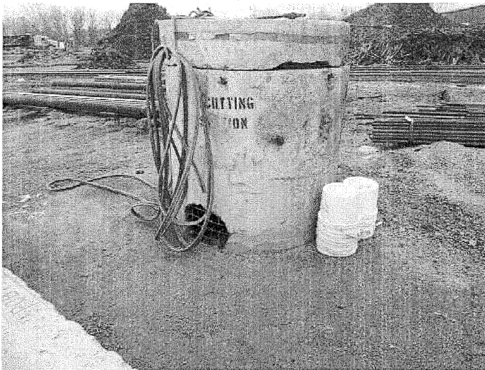
Image 5(Torch Cutting) : One of three torch cutting stations.
