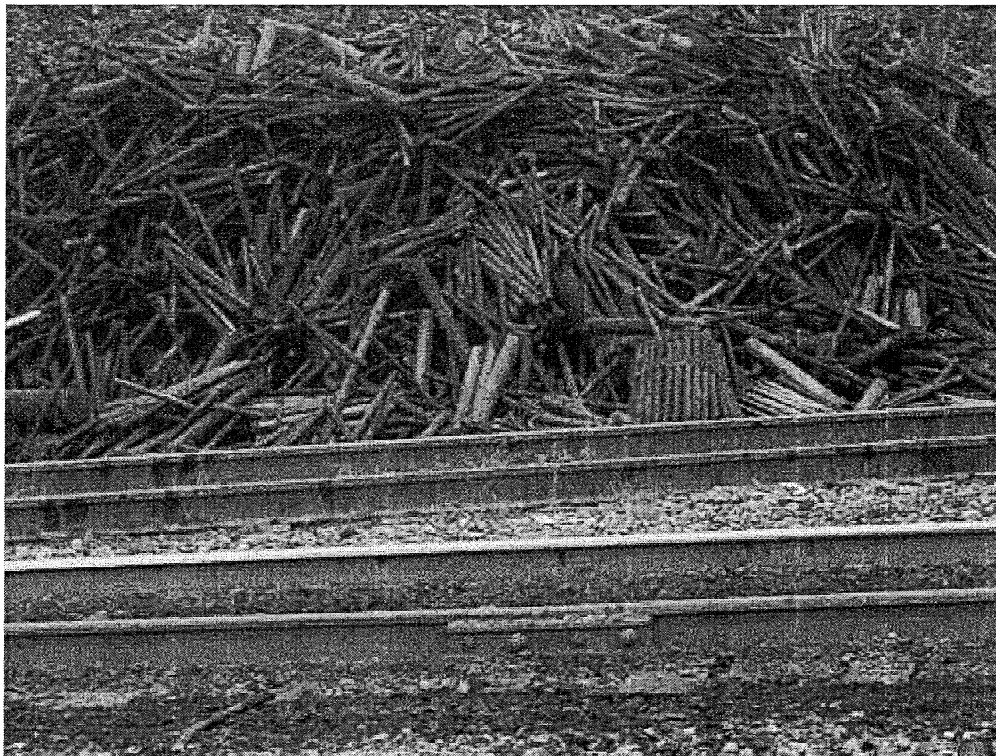
Image 7(Torch Cutting) : Material already cut via torch cutting.
