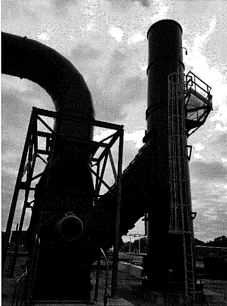
Image 2(New stack-blower) : New stack-blower associated with new castor monovent baghouse.
