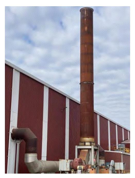
Image 4(Heat treat stack) : Heat treat furnace stack that serves both furnaces.
