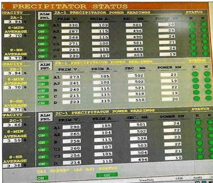
Above are photos of the the ESP operation parameters during my inspection.
