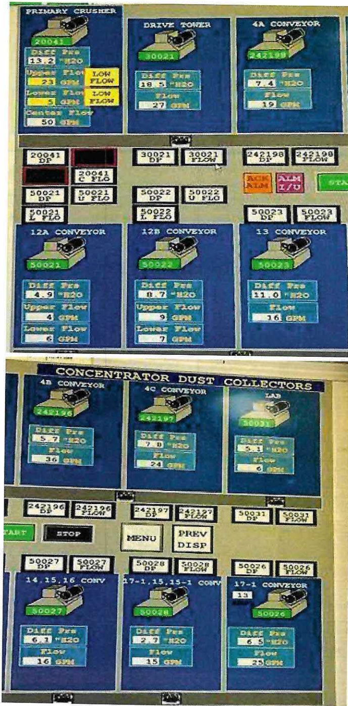
Above are pictures of the operating screen for the concentrator scrubber parameters during my onsite inspection.
