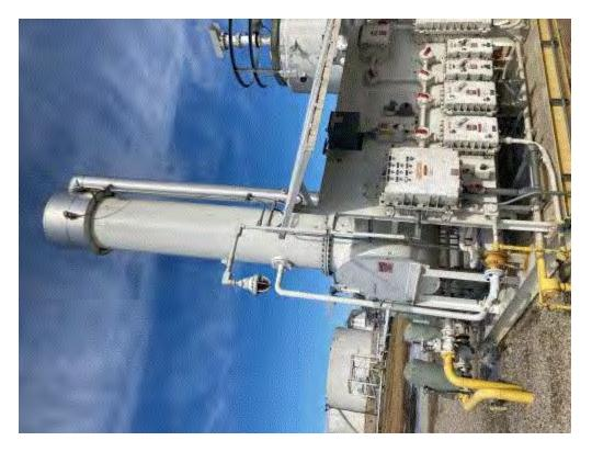
Image 1(VRU stack) : Stack for VOC emissions from VRU carbon bed system.
