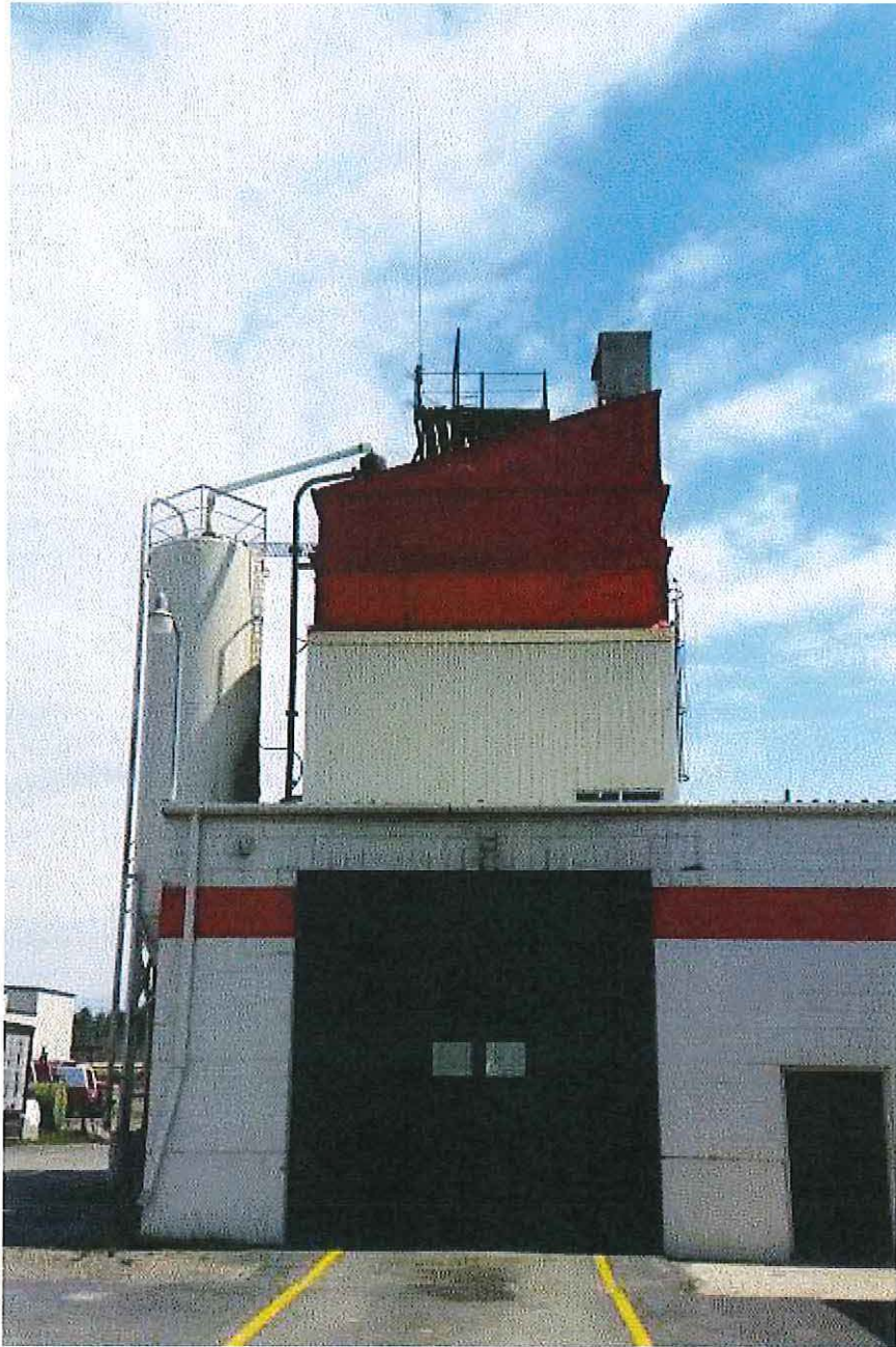
Image 1(MWRM1) : 36-IS Dusty Dustless shaker-style silo filter vent, naturally-vented, positioned on top of load-out area.
