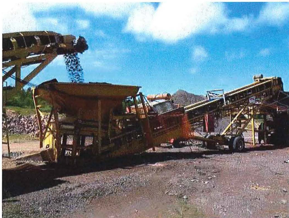
Image 6(SSG5) : T-284 Surge Bin/Conveyor
