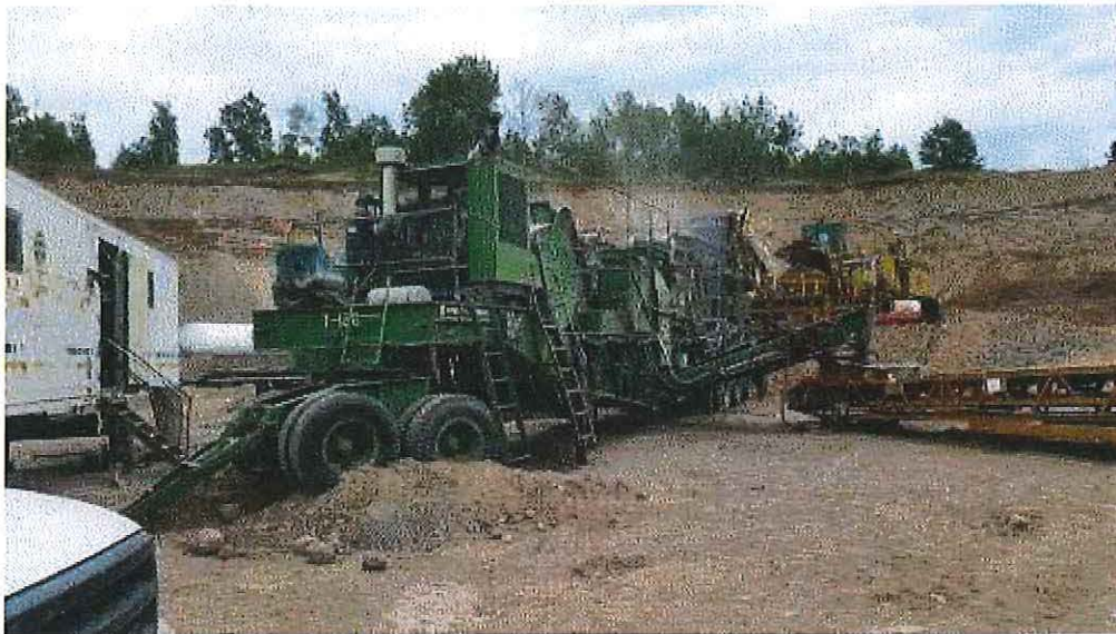
Image 4(SSG3) : Crusher spread
