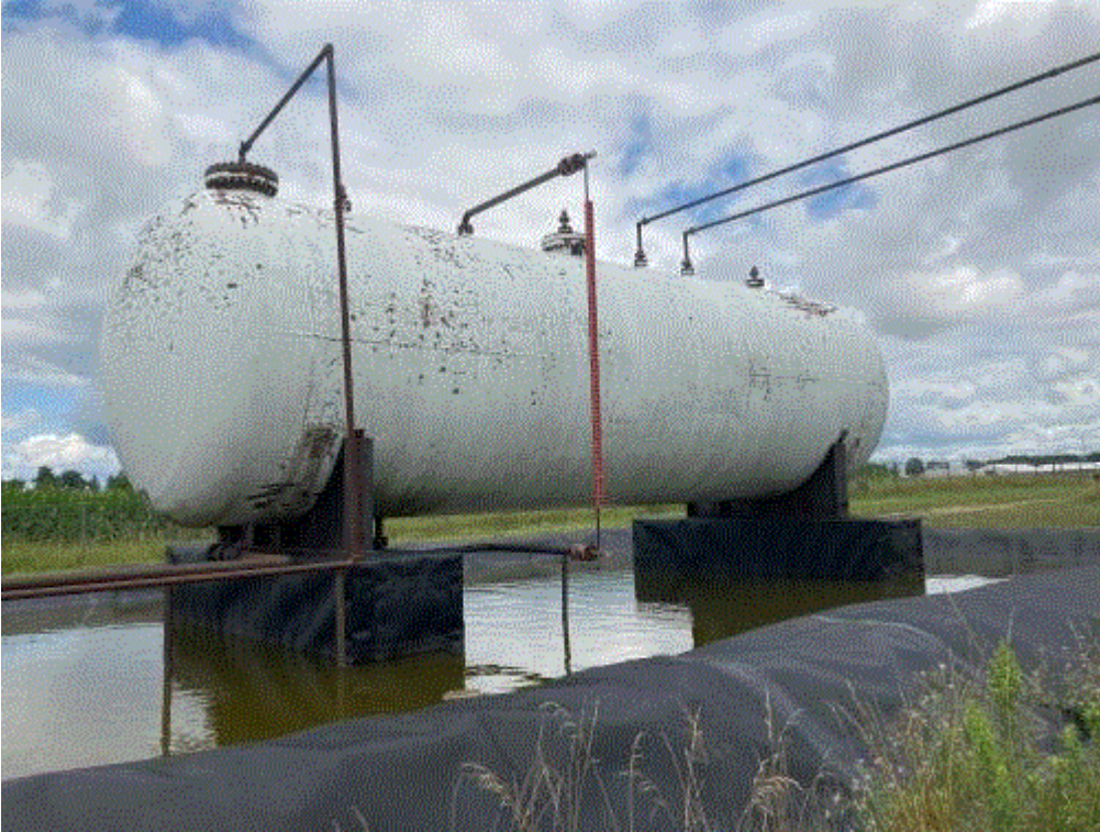
Image 4(NGL Tank) : Shows Secondary containment 1/2 full of water.
