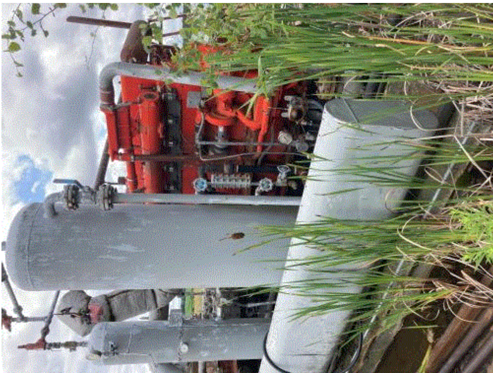
Image 7(Refrigeration Skid) : 6 Cylinder Waukesha Engine
