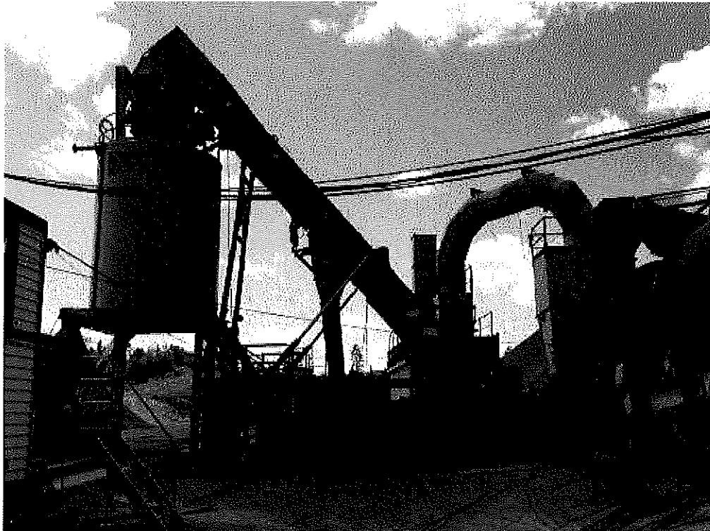
Image 2(B122) : Storage silo w/conveyor for Bacco portable asphalt plant #12
