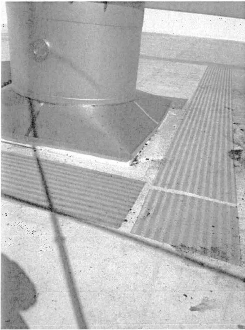
Image 2(Continental roof2) : Base of dryer stack on roof.
