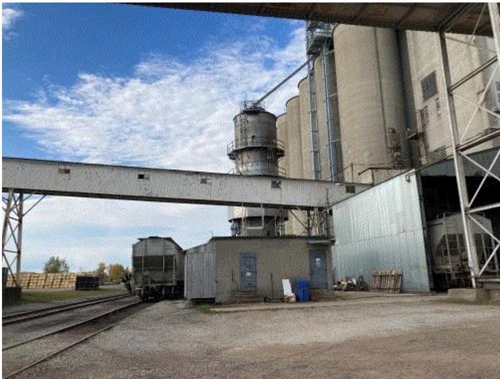
Image 7(Old House Dryer) : View of 3,000 bushel per hour Zimmerman column dryer.
