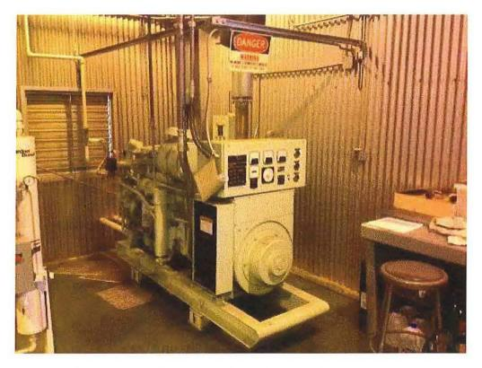
Image 2(GLGT10A2) : Emergency generator APU operates on natural gas
