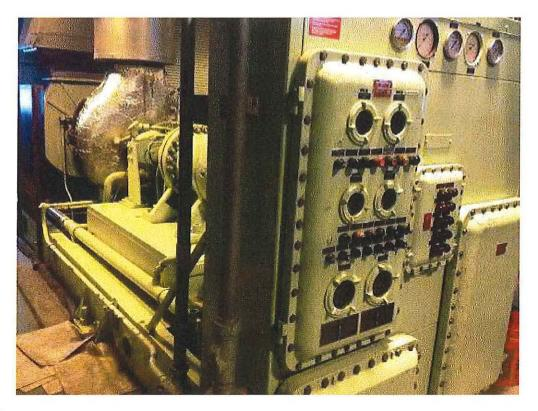
Image 4(GLGT10A4) : Unit 10A02 natural gas turbine pressure generator
