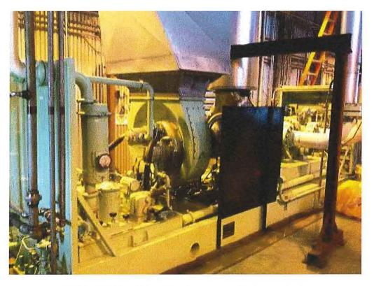
Image 3(GLGT10A3) : Unit 10A01 natural gas turbine pressure generator
