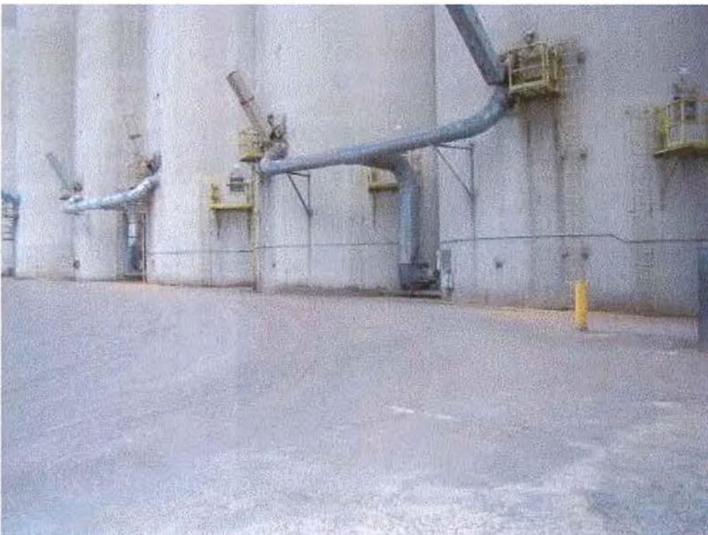
Image 3(Truck load-out spout) : Located on south side of silos. Note minimal beeswings near the silo bases.
