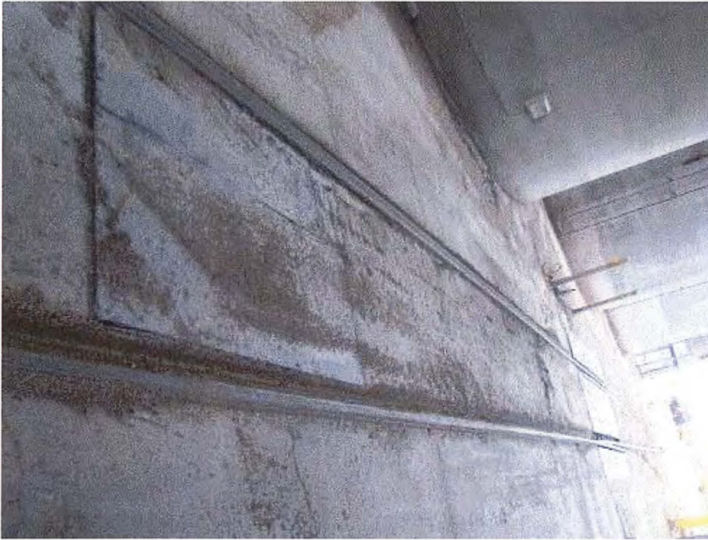
Image 4(Railcar unloading) : unloading pit located underneath the plywood in the middle of the tracks
