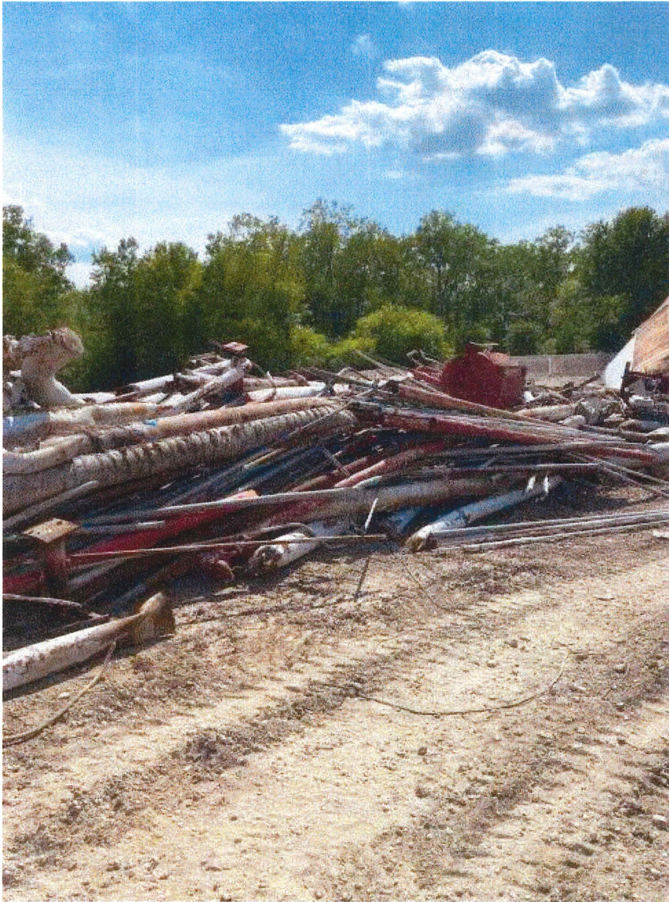
Image 2(Piping) : Remains of the tank piping system after wrecking activity
