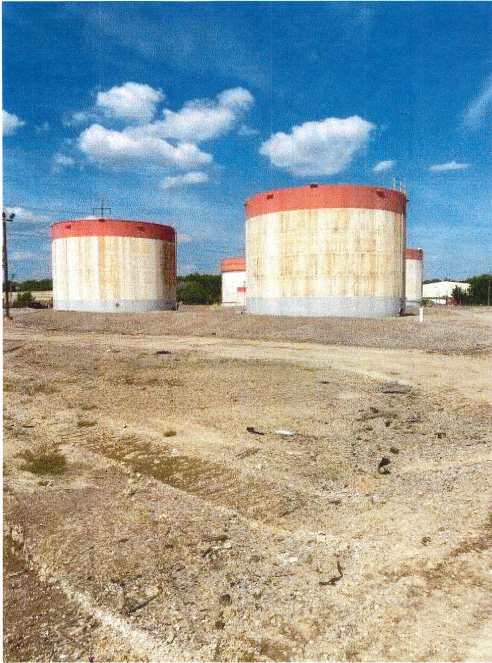
Image 7(Tanks) : Standing Storage Tanks
