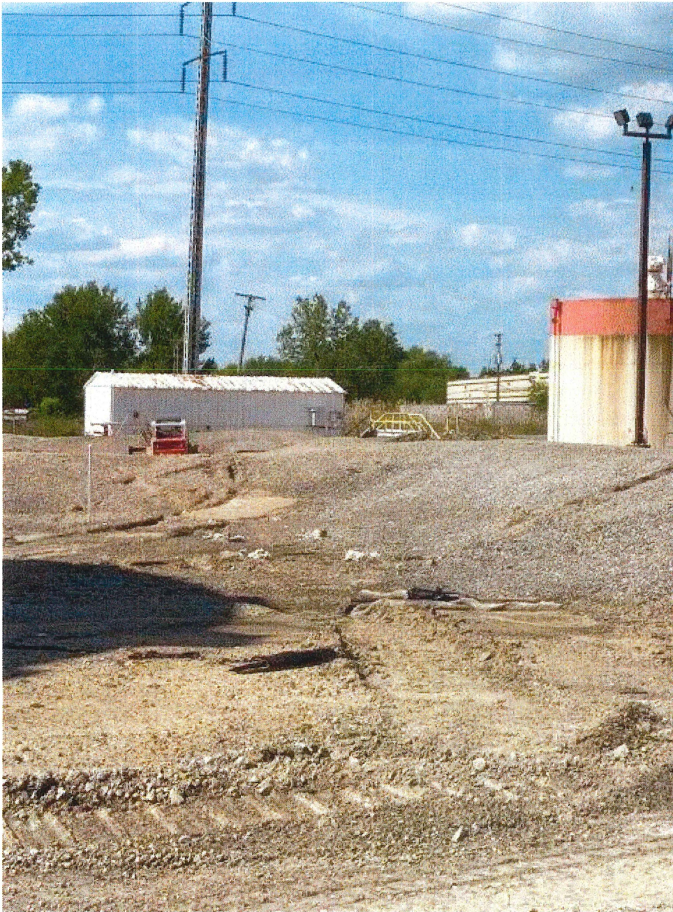
Image 4(Electrical Building) : One-floor Standing Building housing the Electrical Controls and Switches
