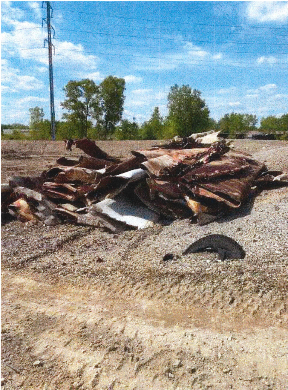
Image 3(Metal) : Metal sheets from dismantled tank
