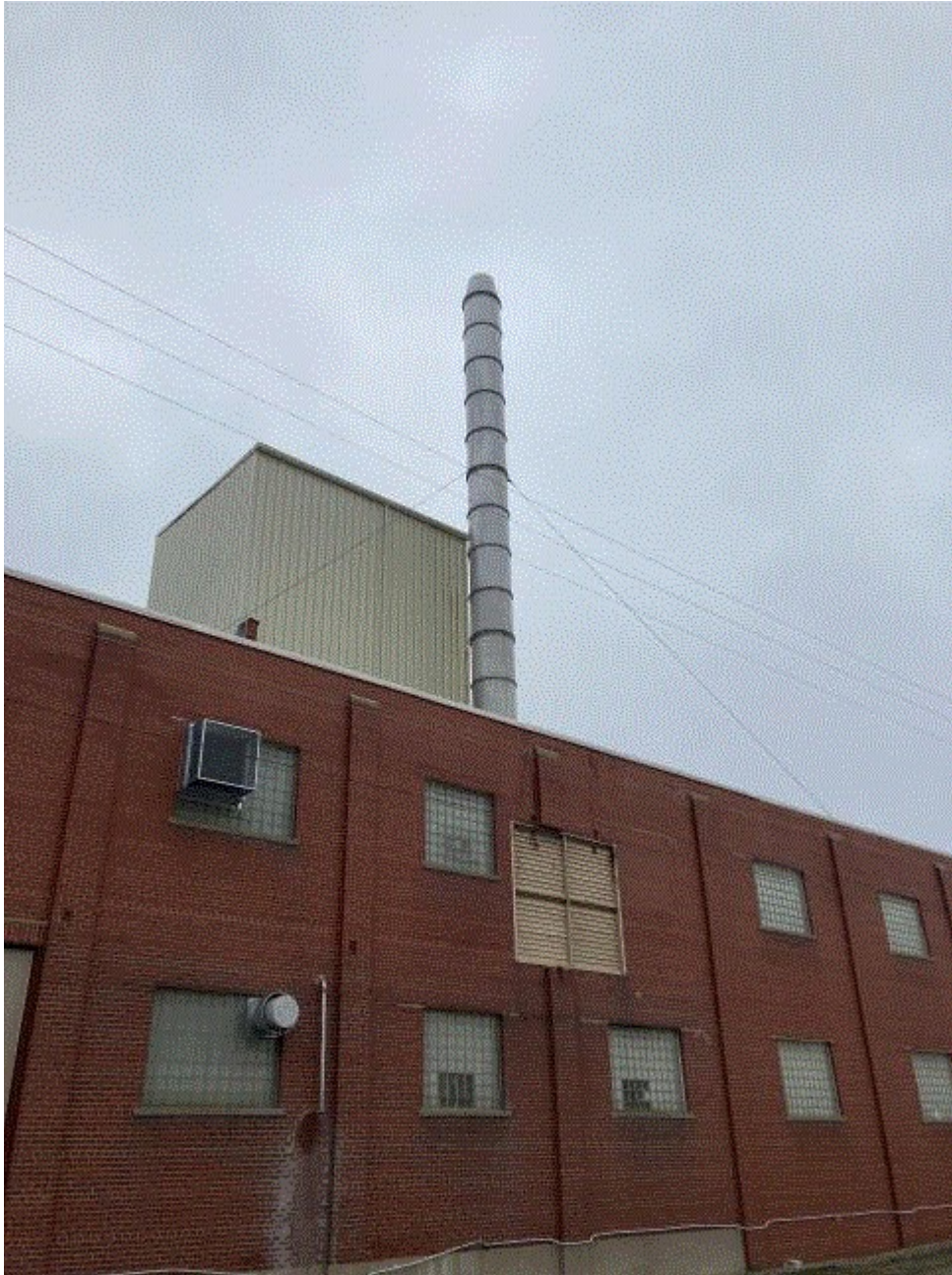
Image 4(Stack) : Close-up view of stack
