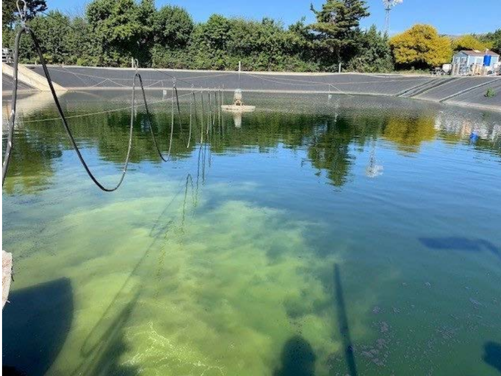
FIGURE 10 INFUSION OF SUPERSATURATED OXYGEN EMULSION
