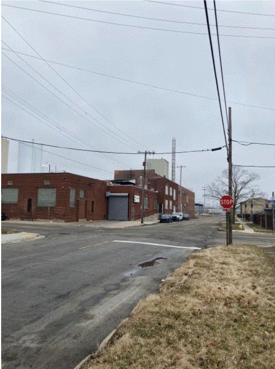
Image 1(Facility view) : Facility view from Church Street.
