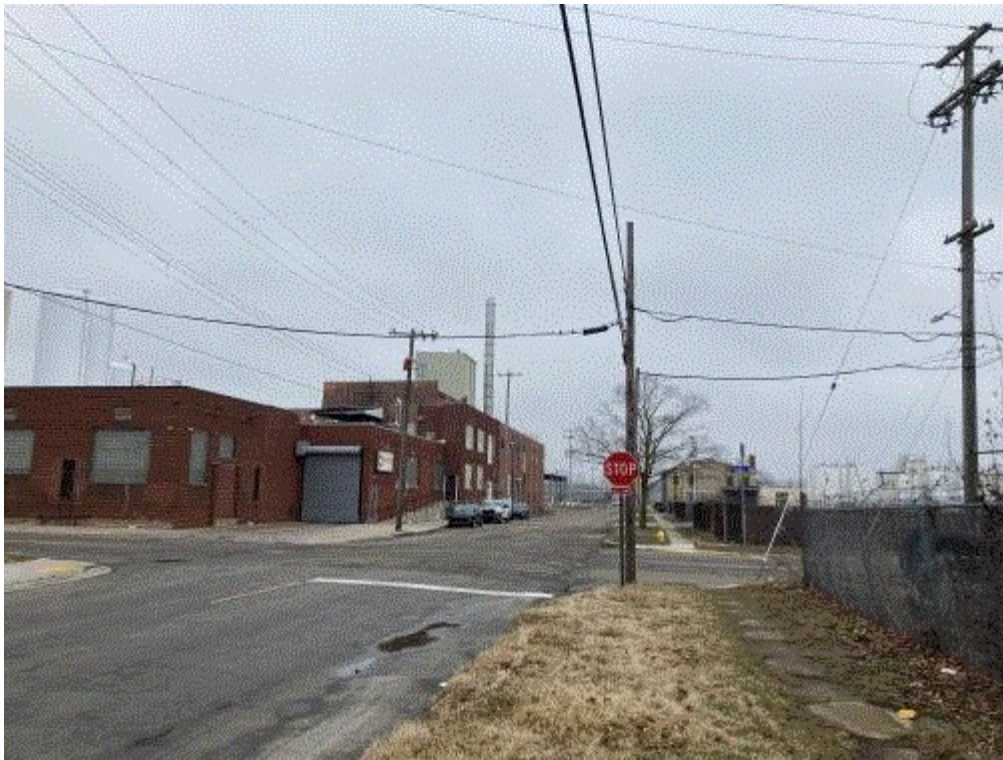
Image 2(Facility view) : Facility view from Church Street
