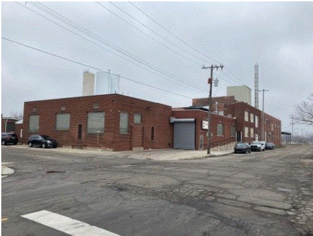
Image 3(Facility view) : View of Facility from corner of Church and Gulf
