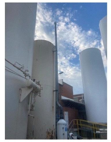
**Image 2(Sludge Tank) :** Photo of the corrected exhaust stack for the sludge tank.
