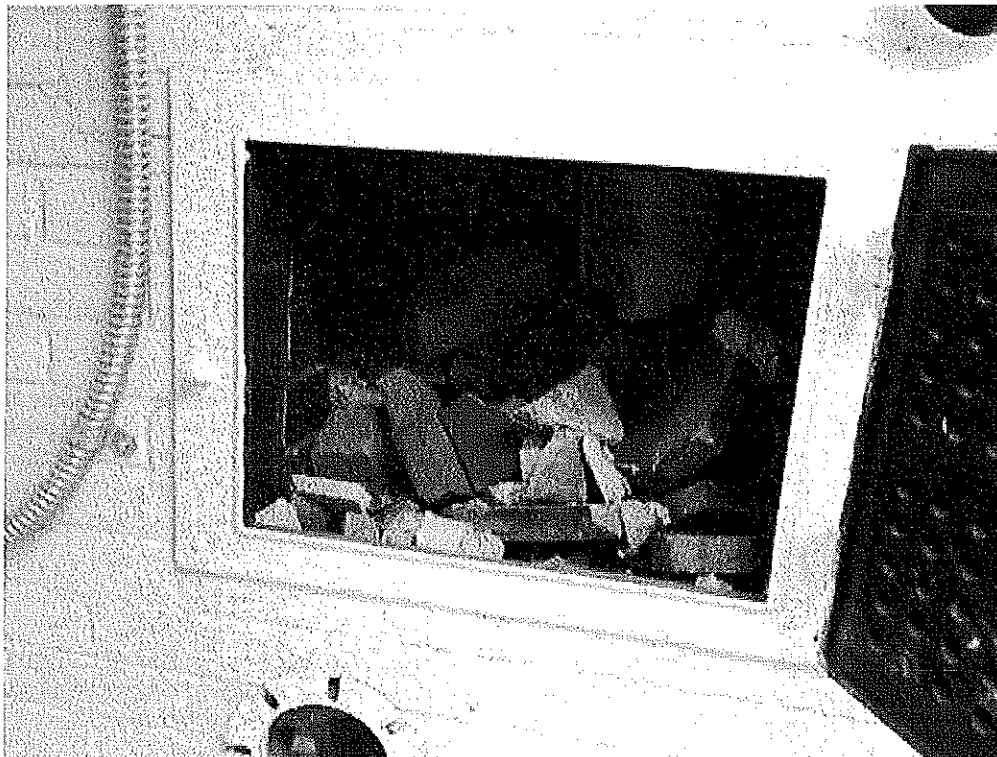
Image 2(incinerator) : Picture of now-closed incinerator, showing remodeling debris that has filled the combustion chamber.
