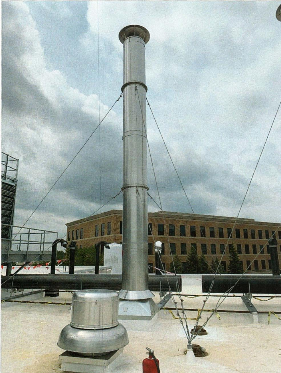
**Figure 3.1:** Example of FGBOILERS (EUBOILER1, EUBOILER2 or EUBOILER3) Sampling Location
