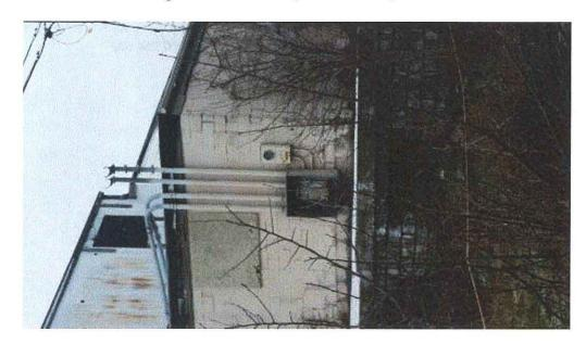
Image 1(Disconnected E Meter): Disconnected electrical meter on south east side of building
