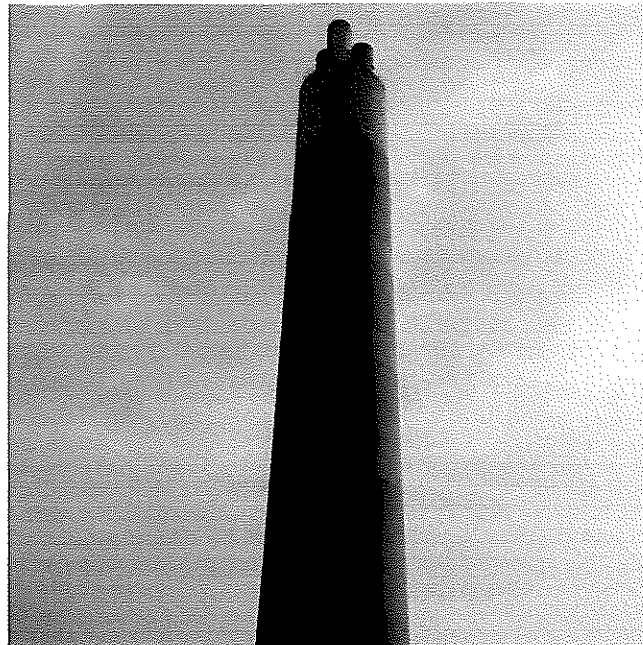
Figure 3.1b: Photo of Stack Exit Point for EUBOILERS011, 012 and 013
