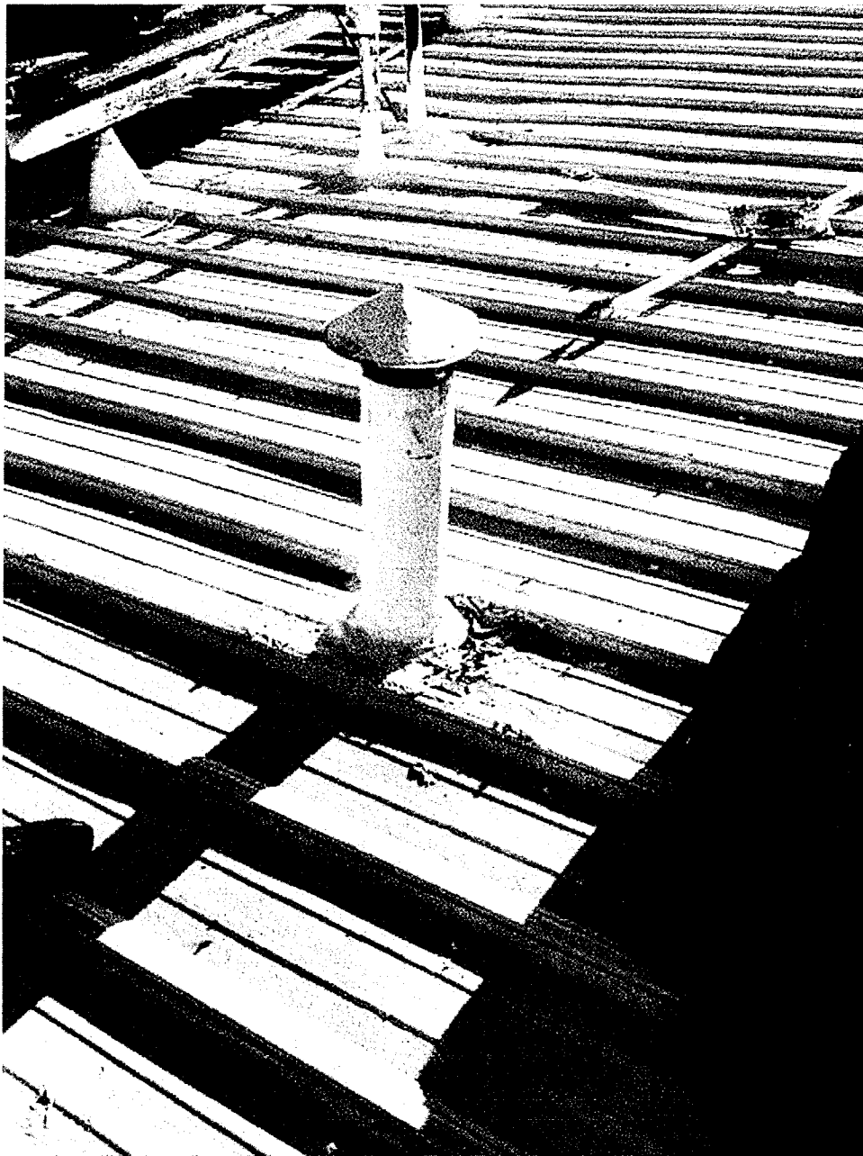
Image 2(Wheelabrator Exhaust) : Photo Cred: Chad DesRocher. Exhaust stack for wheelabrator on top of roof. I did not go on the roof to observe this exhaust point. There appears to be no dust build-up on the roof. Particulate appears to be controlled properly.
