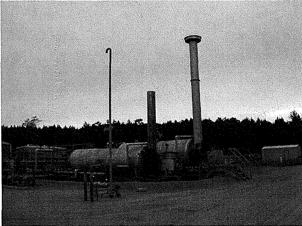
Image 9(inactive heaters) : view of inactive inline heaters located east of the pump house and the crude ASTs and load outs on south side of facility.
