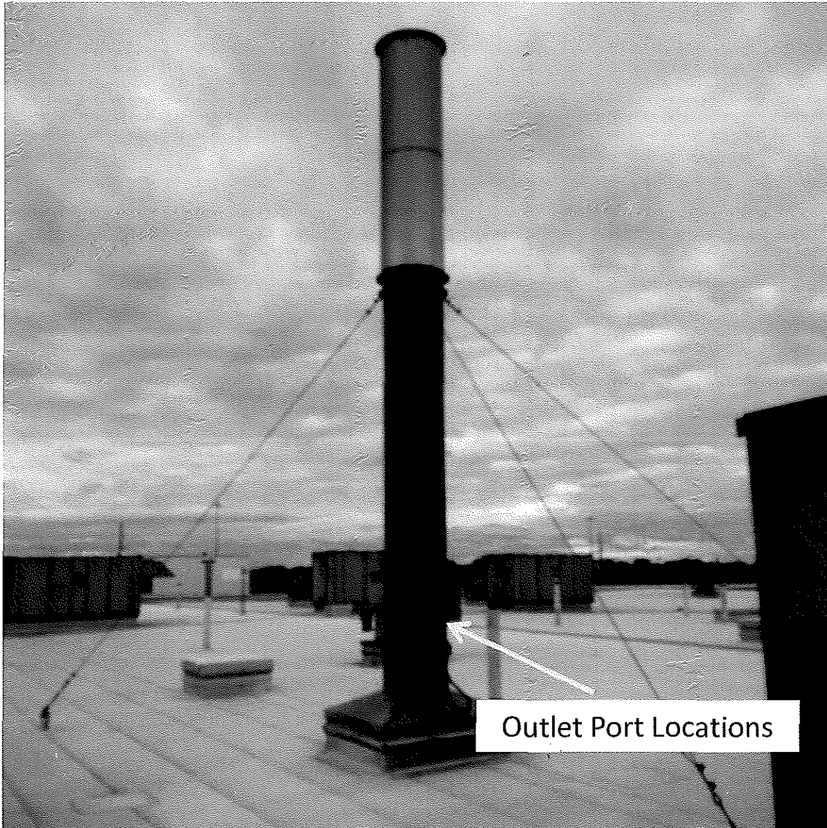
Figure 8: EU-TOPCOAT Oven 1 RTO Outlet
