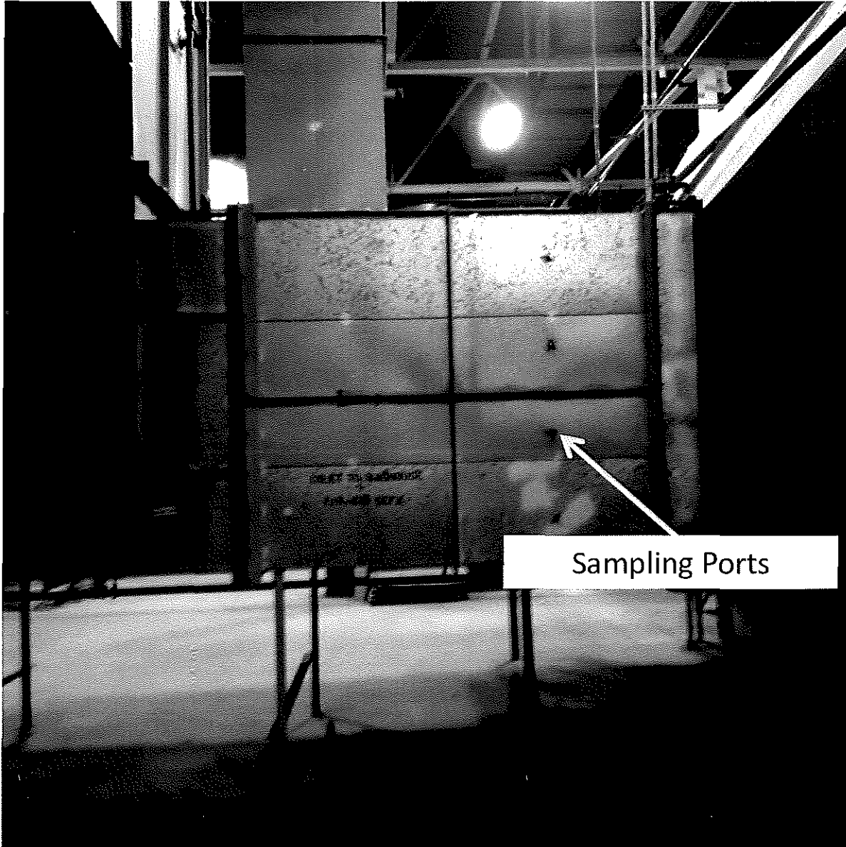
Figure 5: EU-TOPCOAT 3 Concentrator Inlet
