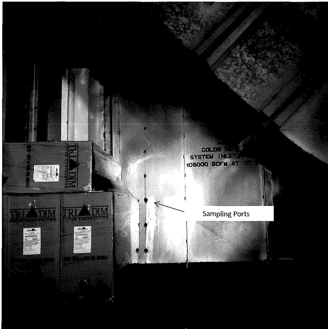
Figure 1: EU-TOPCOAT 1 Concentrator Inlet
