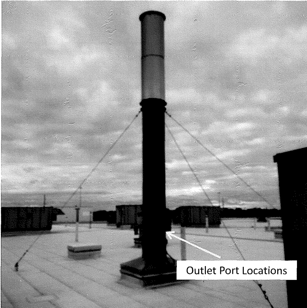
Figure 8: EU-TOPCOAT Oven 1 RTO Outlet
