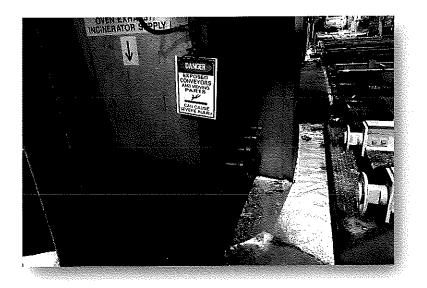
This sampling location is not considered ideal according to U.S EPA Method 1. The outlet location is a 30" x 38" duct with flow disturbances ~4 stack diameter up and ~1 duct diameters downstream of any flow disturbances. This sampling location is considered ideal according to U.S EPA Method 1.
