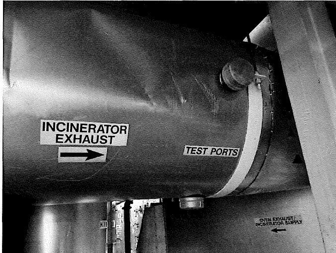
Figure 11: EU-TOPCOAT Oven 2 TO Outlet (THC Sampling Location)
