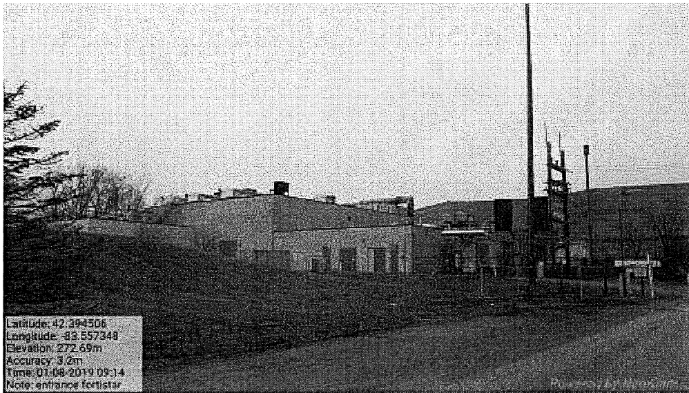
Image 2(Entrance) : Entrance to facility
